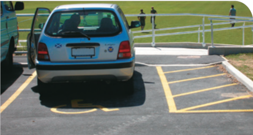
The accessible route to the ramp is clearly defined.
